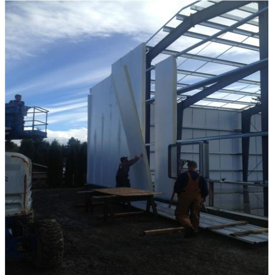
4. Once the first panel is set in the base track it needs to be leveled (this can be done with any method used to keep the metal panels on module – Laser level, carpenter's hand level, etc.) Periodic checks need to be made as the panel is installed to ensure that it is staying level as it is going on down the wall.
