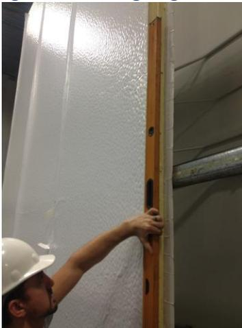
6. Once the bottom of the panel is locked in tight, push on the leading edge of the panel to make sure the top is locked in tight at the same time as you are pushing the panel into the wall to stick it to the girt with tape on it.
