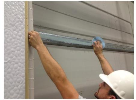
3. Stand panel on the wall. In most cases one person can stand the panel on walls under 25' eave height. The best method for standing the panel is to put the bottom of the panel up against the base track and walk the panel up as seen below.
